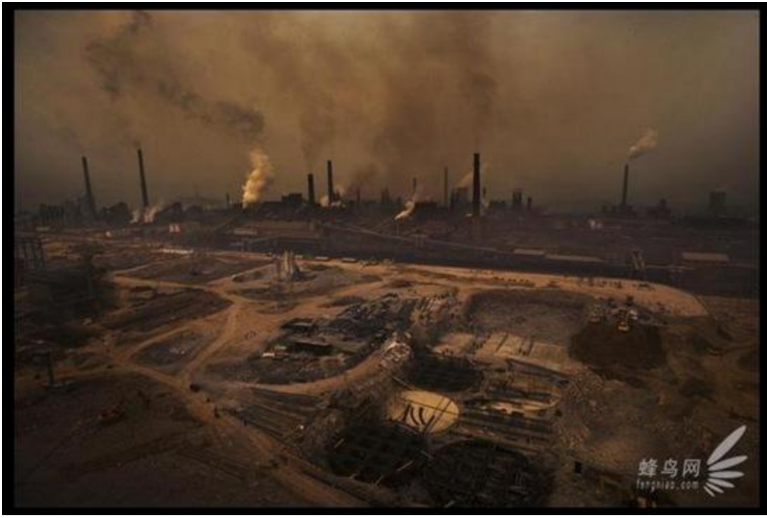
Shexian Iron and Steel plant, Hebei province. March 18 th , 2008.
